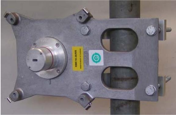
A photograph showing a silver metal remote mount kit (RMK) attached to a dark metal pole. The RMK has a central circular waveguide interface, several mounting holes with screws, and a yellow label with the text 'RMK1B-2010R'. A green circular logo is also visible on the metal surface.
