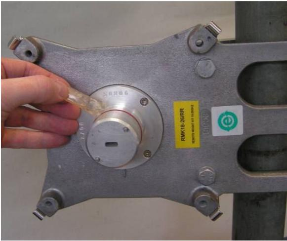
A close-up photograph of a hand applying a clear, viscous substance (silicone grease) from a small tube onto the circular waveguide interface of the RMK. The RMK is mounted on a pole, and the yellow label and green logo are visible in the background.
